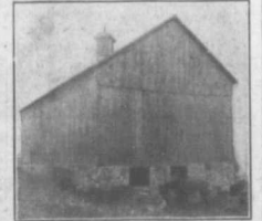
Barn as shown above, 56 by 30, on stone foundation, stable for three horses, 6 cows and about 10 pigs, henhouse, root cellar, well under the barn for stock.
