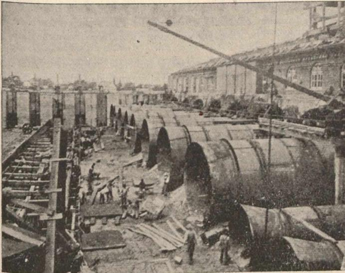
Fig. 3.—Setting the Penstock Tubes.
