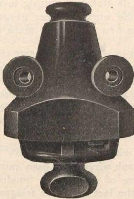
Transformer Primary Cut-out.—Showing insulator top, holes for screws and openings for viewing fuse.
