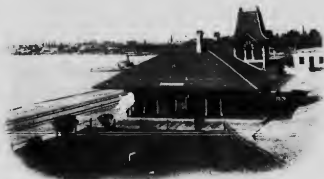
Grand Trunk Railway Station Barrie.
