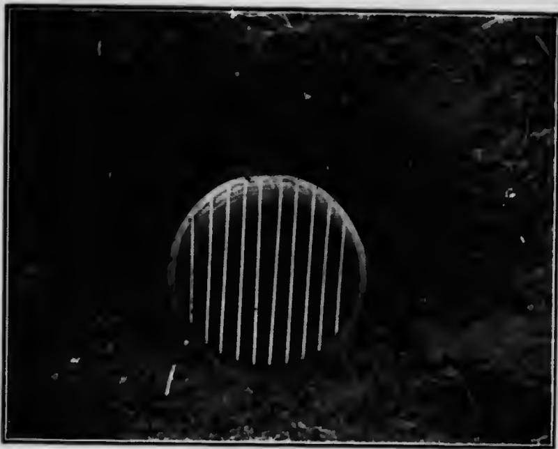
Fig. 21. End view of corrugated metal outlet.
