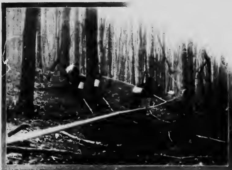
FIG. 9. THROUGH METAL PIPES THE SAP FLOWS FROM THE BUSH TO THE SUGAR HOUSE
