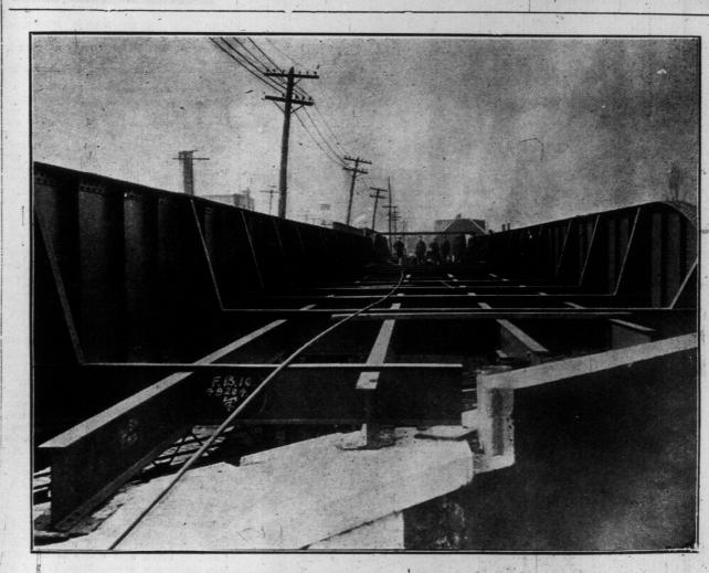
DUNDAS-STREET BRIDGE NEARING COMPLETION. Picture shows entire length of bridge and skeleton of steel beams and girders and gives some conception of the strength of the structure.
