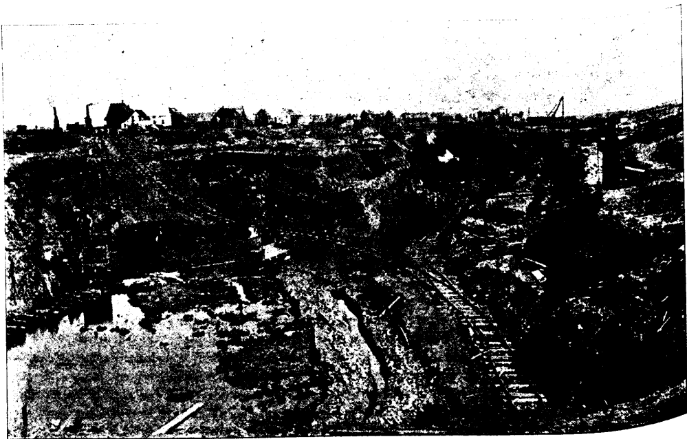
AT FORT LAWRENCE.—EXCAVATING FOR THE CHIGNECTO SHIP RAILWAY.
