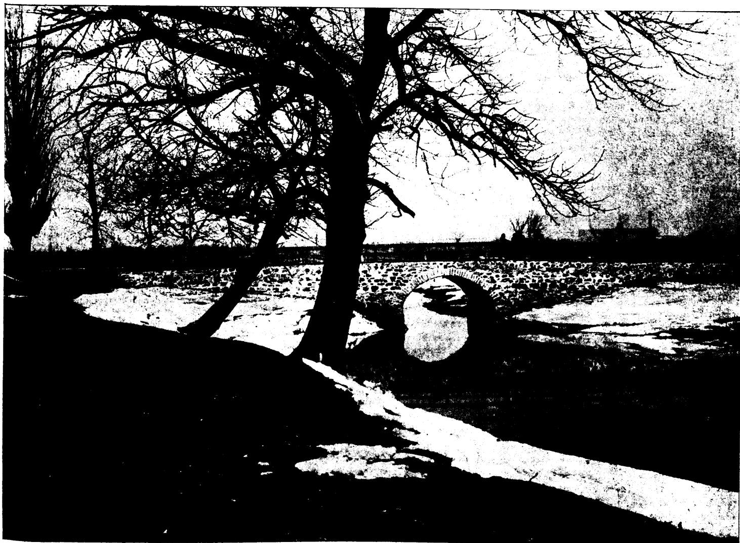
ON THE LOWER LACHINE ROAD. (Bridge over the St. Pierre River.)
