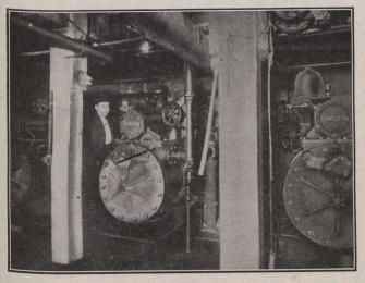
Special pump chamber arranged to one side of shaft at depth of 300 ft. Equipped with three horizontal Cameron pumps.
