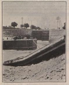
Fig. 3. Lower Gates of Lock 22, Replaced.
