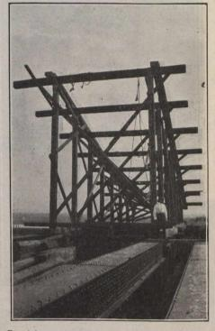
Derrick erected to assist the Floating in of the 408 ft. spans, C.P.R. Lachine Bridge.
