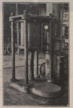
Air Press with Double Reading Gauge for Testing Coach Springs.
