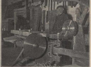
Fig. 3-Tie Plug Forming Machine Cutting off Finished Plugs.
