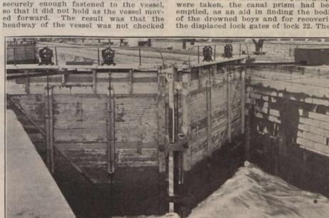
Fig. 6. Gowan Safety Appliance on a Lock Gate.
