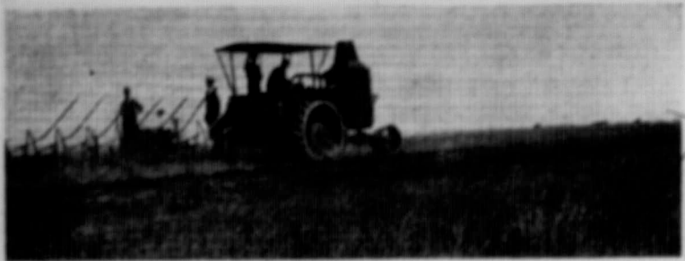
KEROSENE TYPE OF ENGINE AT WORK WITH TEN BOTTOMS
