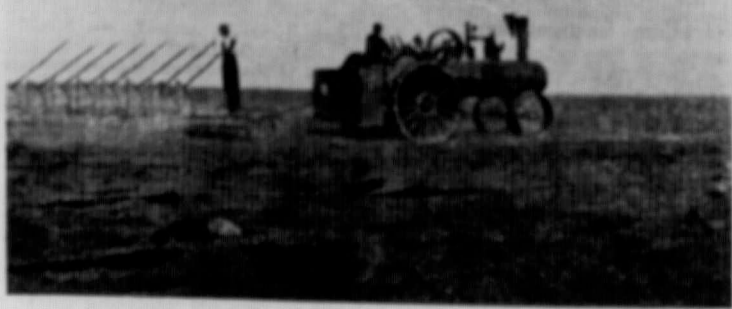
60 H.P. STEAM ENGINE BREAKING WITH 8 BOTTOMS
