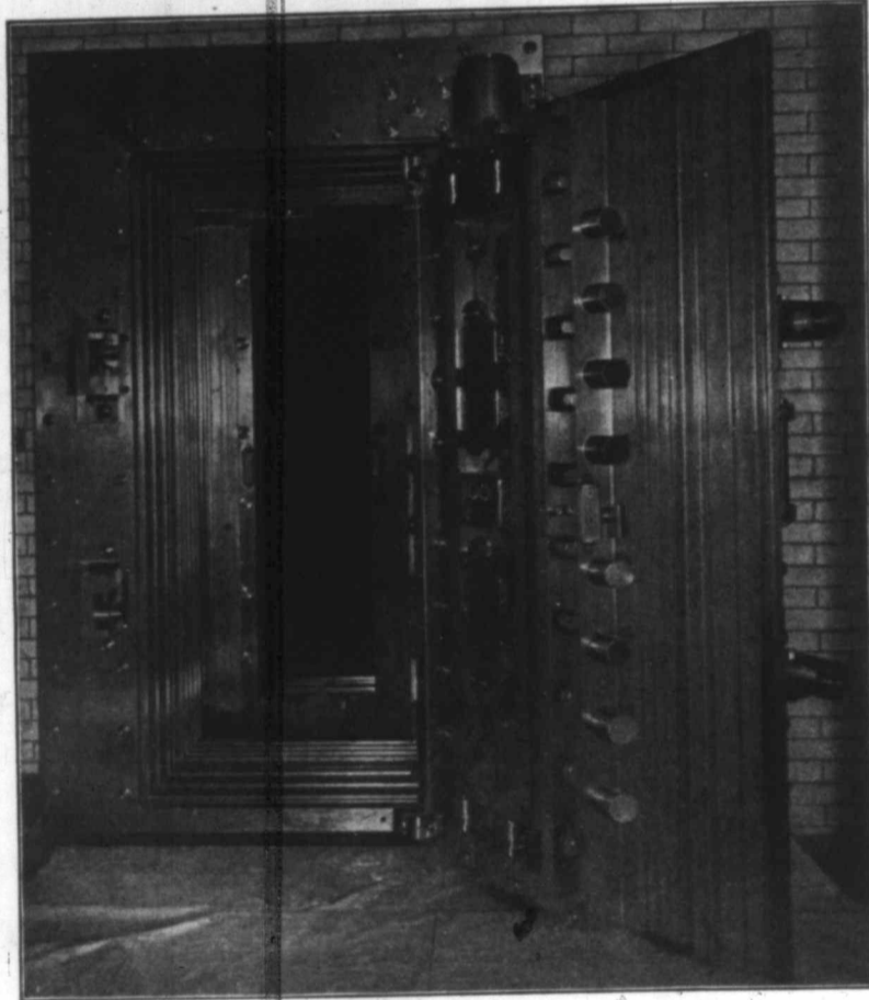
Vault doors in Bank of Montreal and Royal Trust Company, Montreal. Three times larger and heavier than any other in Canada. Doors and Vestibules weigh 60 tons . Total weight of lining and doors 260 tons . Accepted to be the finest piece of vault work in construction and workmanship in the Dominion. — Built by the old established firm of
