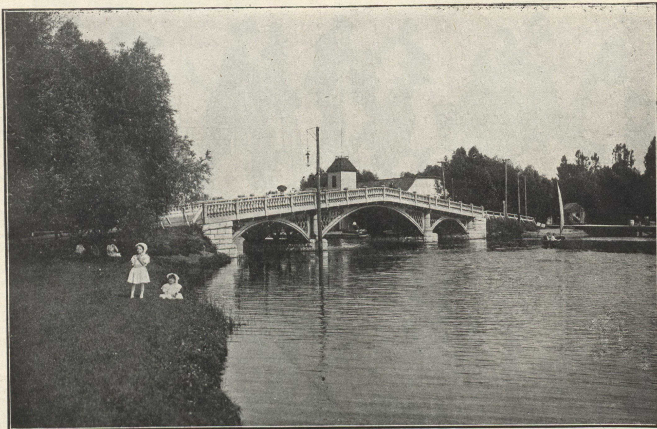
Bridge Crossing Lagoon, Island Park.
