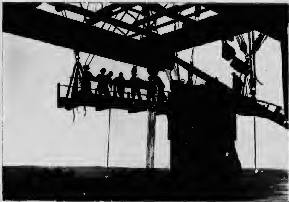
DRIVING A 12-INCH TOP CHORD PIN.
