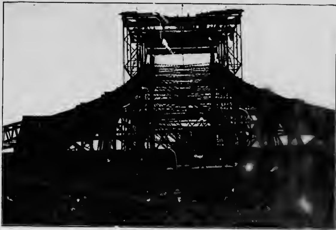
VIEW OVER TOP OF SOUTH ANCHOR ARM.
