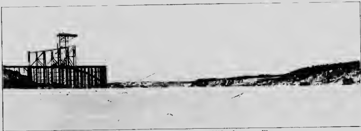
THE WORK AT THE END OF SEASON OF 1903. LOOKING WEST.
