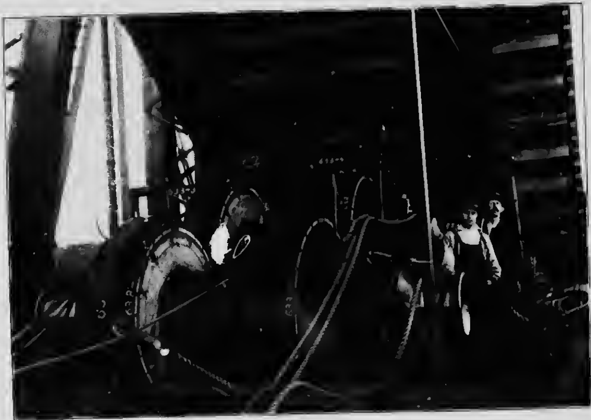
ONE OF THE 125-HORSE-POWER HOISTING ENGINES.
