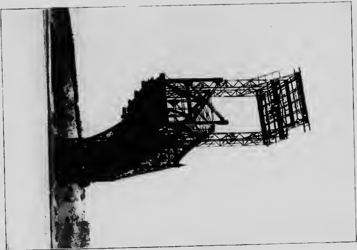
SOUTH CANTILEVER ARM FROM RIVER.
