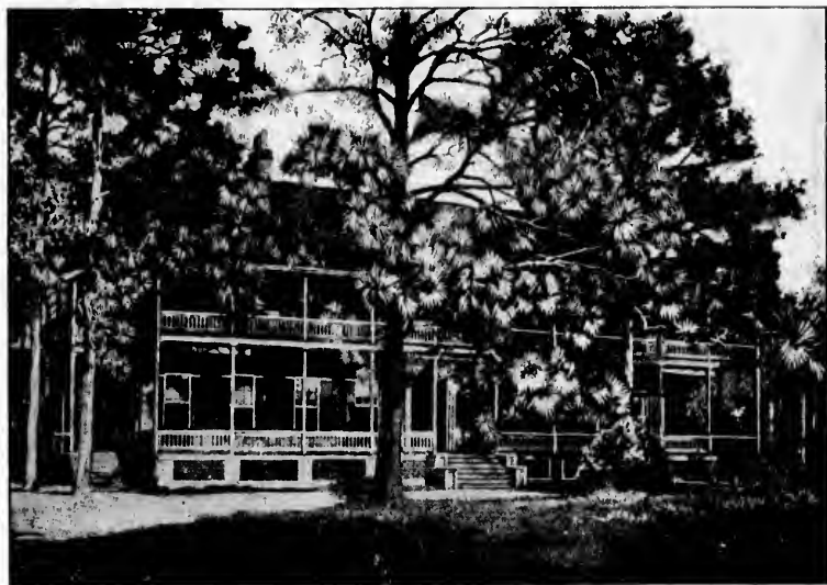
FIG. 58.—MAIN BUILDING OF THE SANATORIUM HYGEIA AT CITRONELLE.
