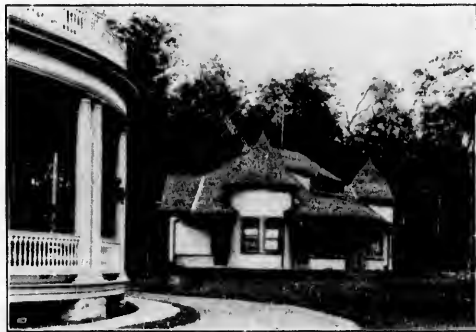
FIG. 62.—A COTTAGE OF MUSKOKA COTTAGE SANATORIUM.
