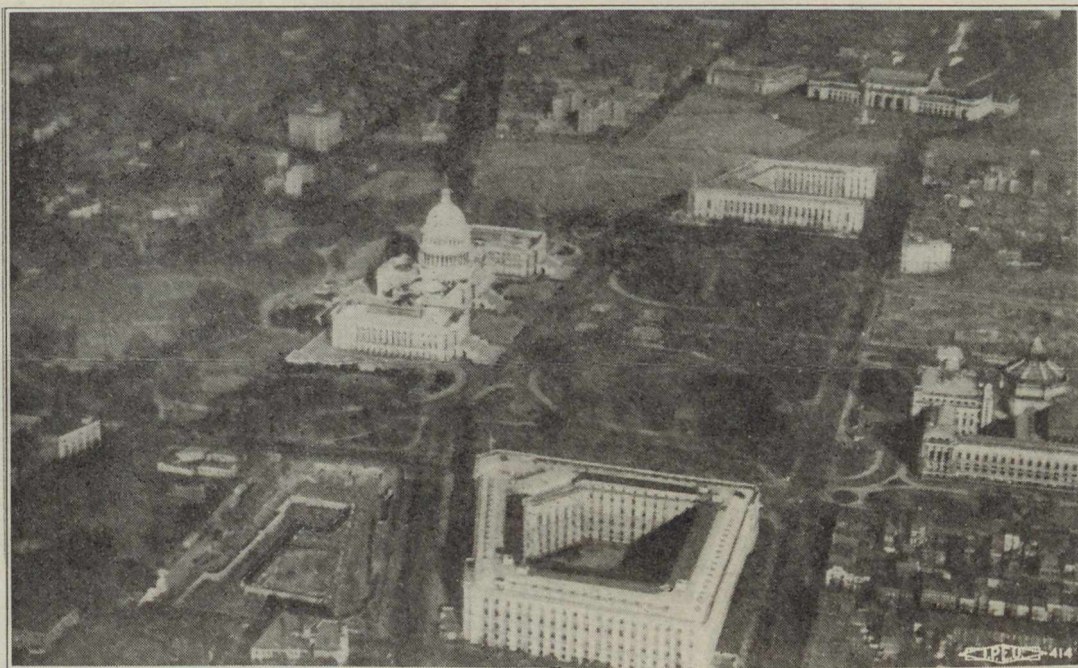
THE NATIONAL CAPITOL AND ITS SURROUNDINGS VIEWED FROM THE AIR
