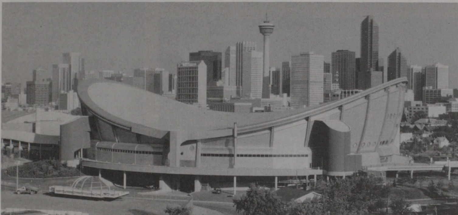
Calgary, Alberta, with the Olympic Saddledome in the foreground.
