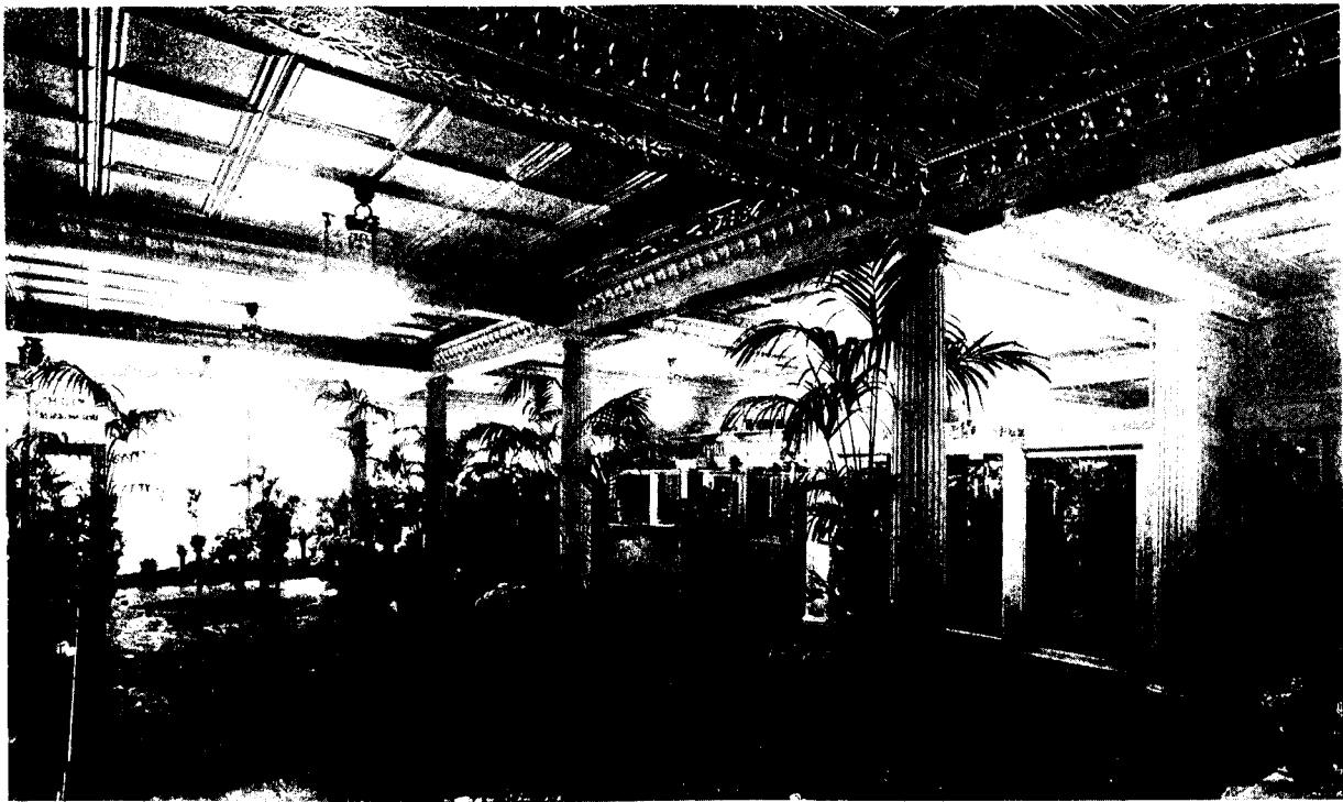
Interior of New Store of Dunlop the Florist, Toronto. Contractor—James Gow.
