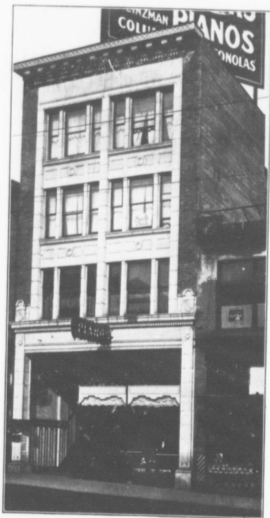
New premises of Fletcher Bros., Ltd., Vancouver, B.C.
