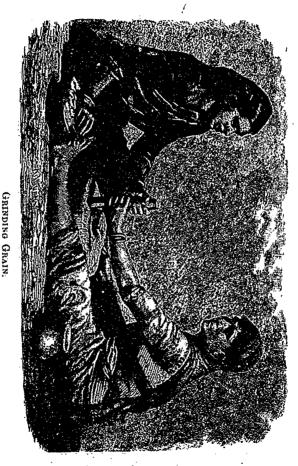
another hole in the centre, through which the grain passes and is ground by turning the upper stone upon the lower one.
