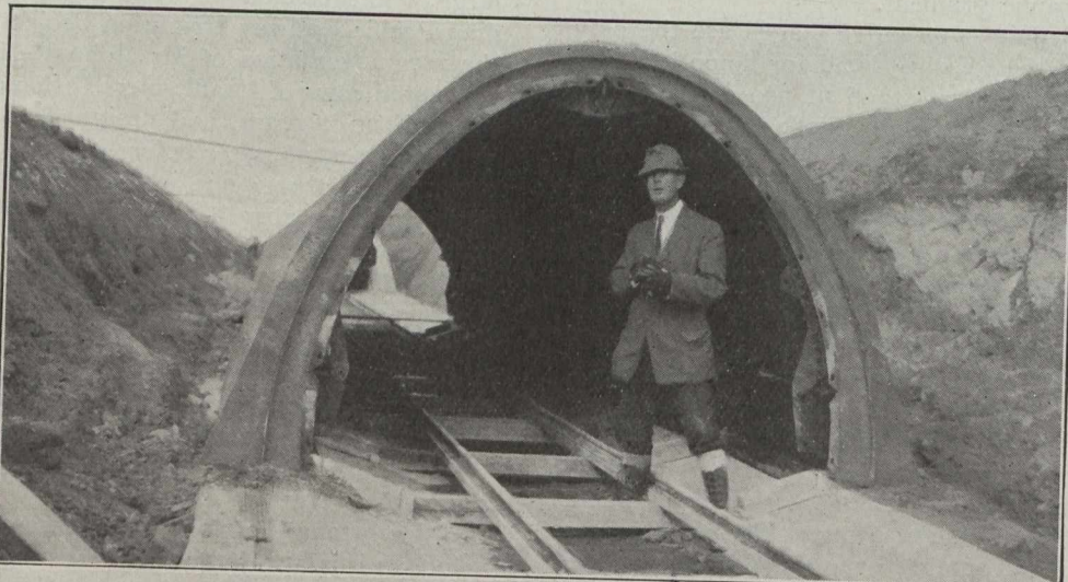
Fig. 3. Concreting Closure Arch Between Alternate Sections.
