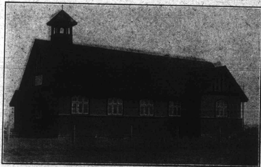
ST. STEPHEN'S CHURCH, WINNIPEG.
