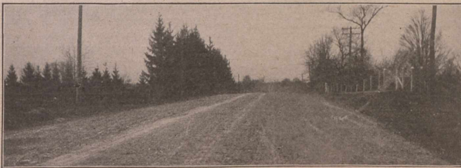
A GOOD GRAVEL ROAD—But with a Wider Grade than is Necessary—County Wellington
