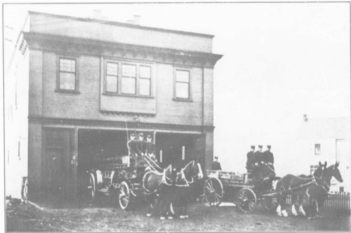
No. 10 FIRE HALL, Thirteenth Avenue and Heather Street.
