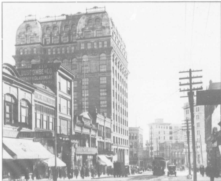
Hastings Street, showing a few modern Office Buildings.
