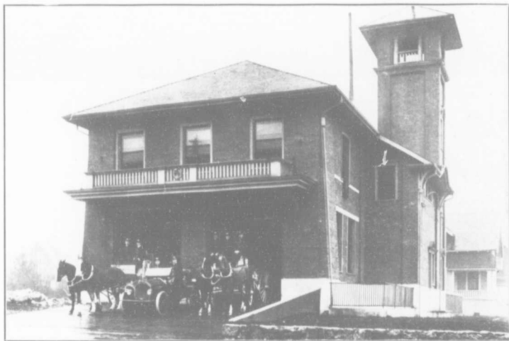
No. 9 FIRE HALL, Salisbury Drive and Charles Street.
