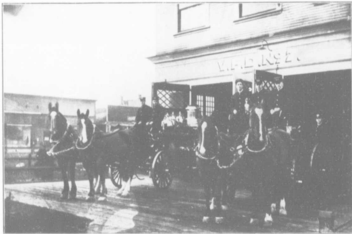
No. 7 FIRE HALL, Corner Fifth Avenue and Yew Street
