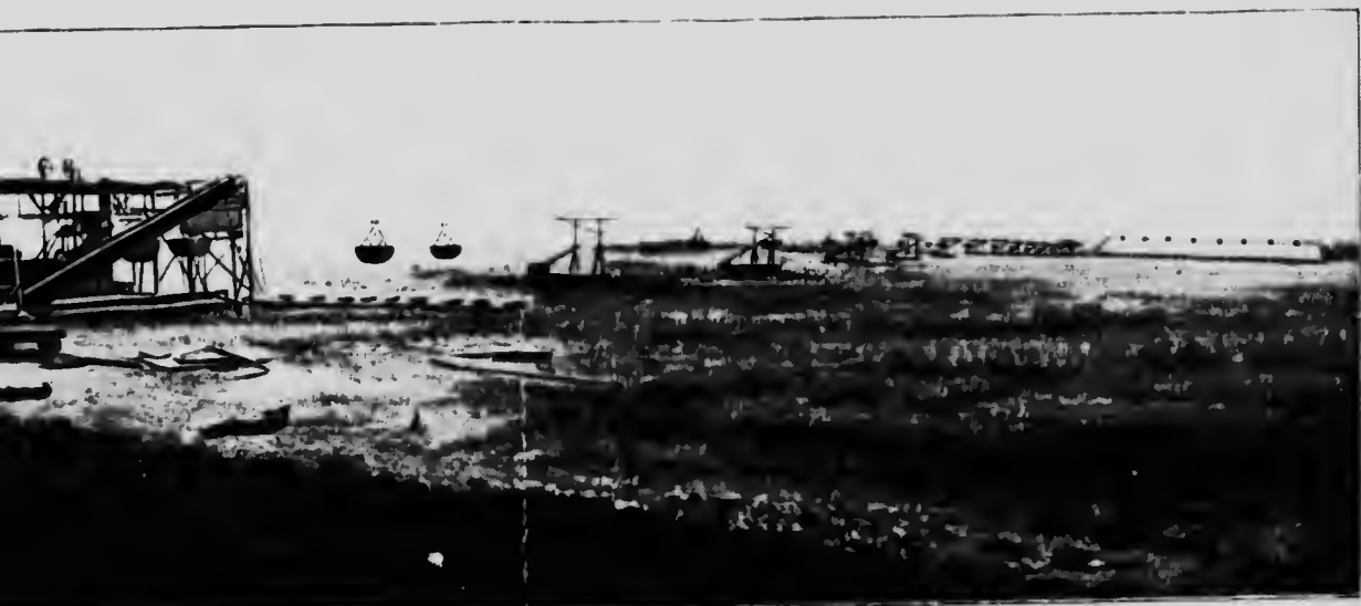
's cable device for transportation of raw peat fuel, at the Alfred peat bog, Ontario.
