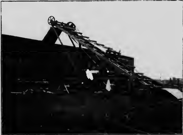
Elevating system. Loading dry peat into railway cars at Alfred, Ontario.
