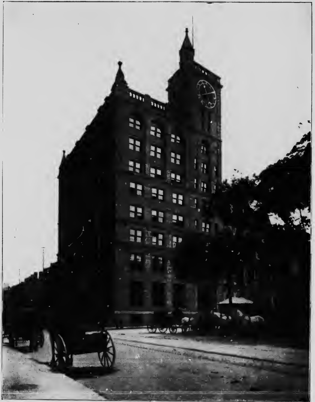
New York Life Insurance Company Building, Place d'Armes Square and St. James Street Montreal.
