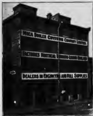
Montreal Factory and Warehouse
