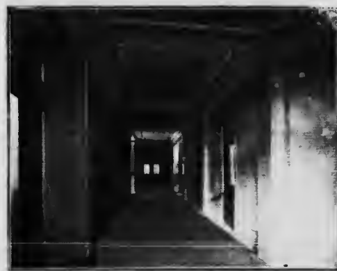
Corridor in Coristine Building.
