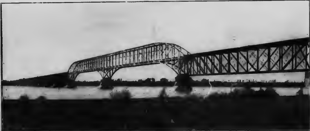
St. Lawrence River Bridge, C. P. Ry., Lachine, P.Q. Built 1886.
