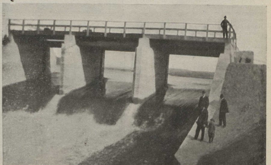
Spillway of the Power Dam Now Almost Completed.
