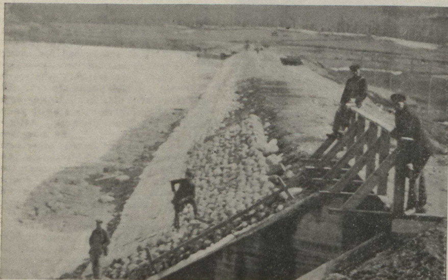
Intake and Dam of the Minnedosa Power Company at Minnedosa, Man.
