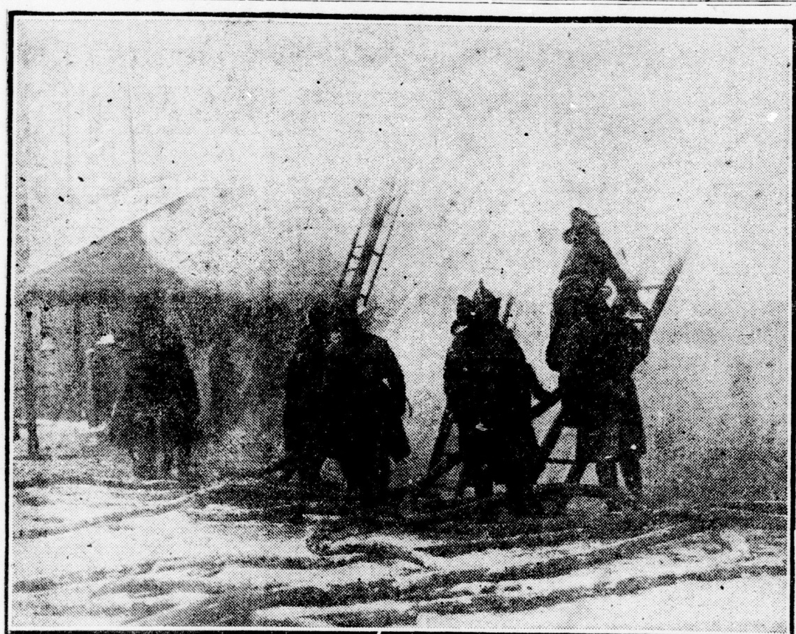
Fire in icy January weather, did $50,000 damage to the Cosgrave
