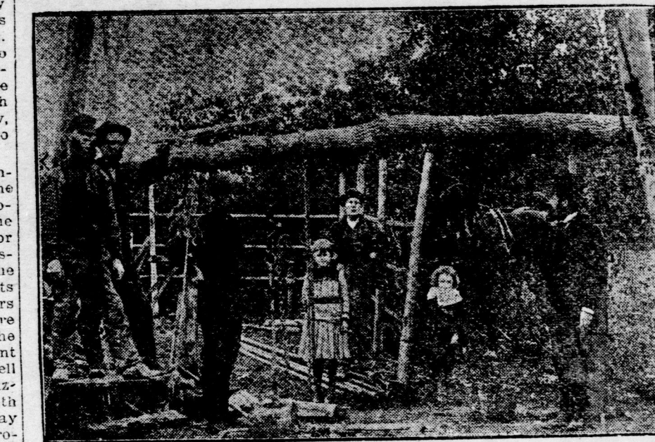
ORIGINAL METHOD OF KICKING A WELL DOWN.
