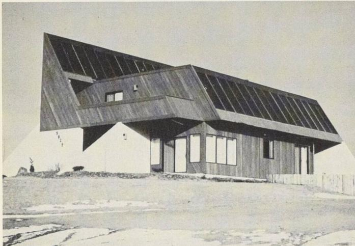
A two-storey demonstration home in Colorado Springs, Colorado. With an 810-square-foot array of collectors (liquid heat transport and storage) at least 80 per cent of this home’s heating demand can be met through solar energy. Supplementary heating and summer cooling is provided by a heat pump.
