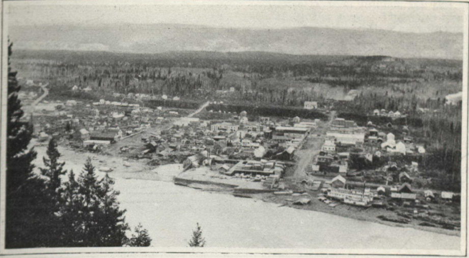
SOUTH FORT GEORGE, ONE OF THE NEW BRITISH COLUMBIA TOWNS
