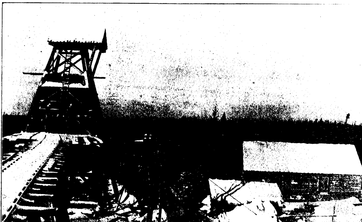
THE FOLEY MINE—DUPLEX HOIST AND TRAMWAY.
