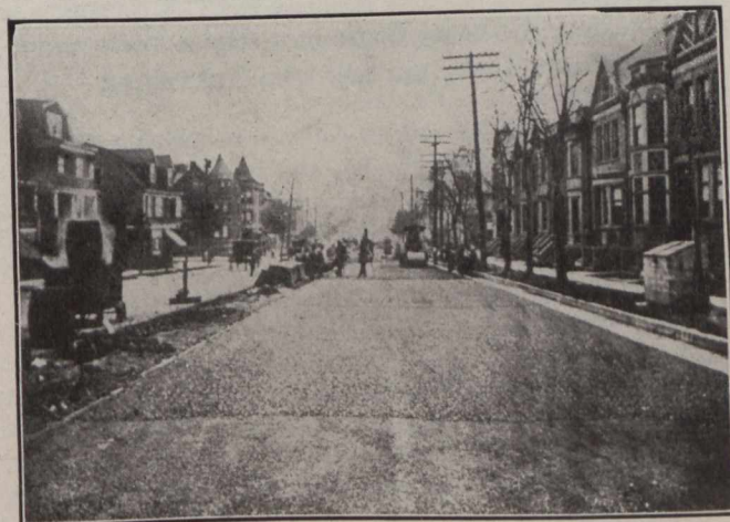
Fig. 3.—Rolling a Tarviated Macadam Road Constructed by the Mixing Method.
