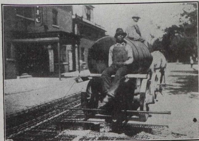
Fig. 2.—Distributing Tarvia "B" by Means of an Ordinary Watering Cart Fitted with a Distributing Device.
