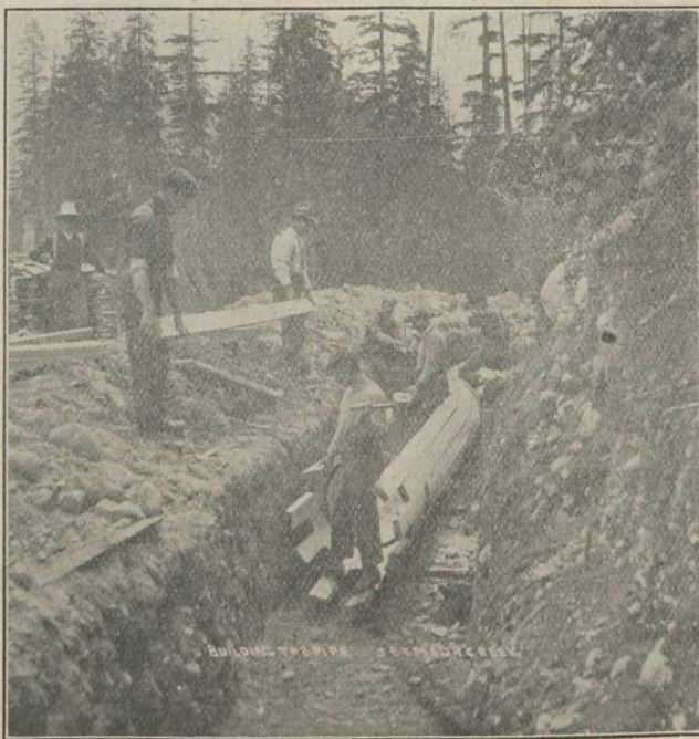
Building the Pipe in the Trench.
