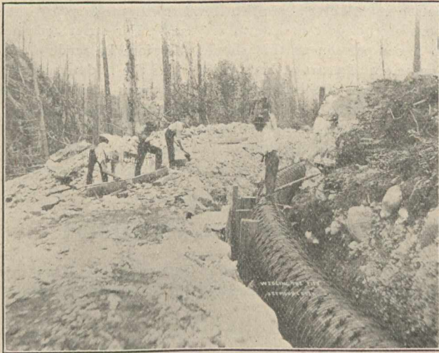
Wedging tee Pipe at a Curve.
