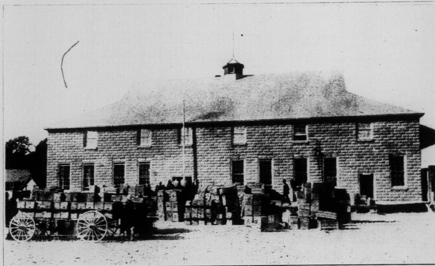
Plant of Old Homestead Canning Co., Picton, Ont.
