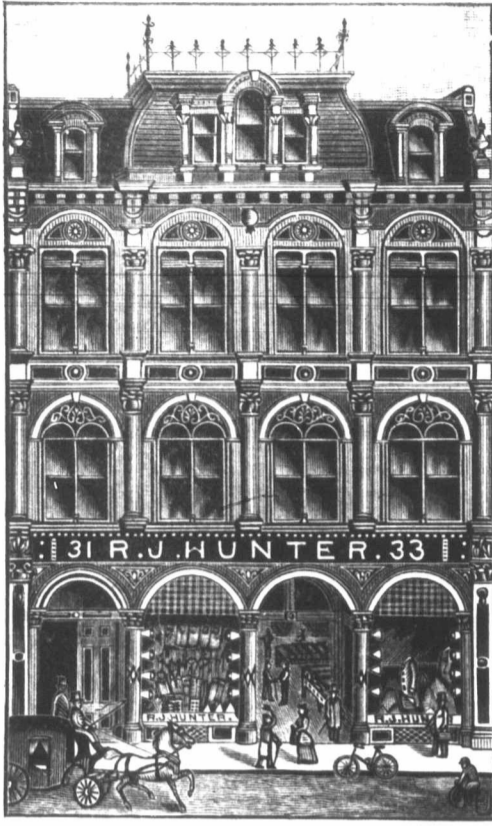
The above cut shows our new premises, 31 and 33 King Street West.
