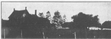
The Pleasant Home and the Farm Buildings on a Prize Winning Farm
