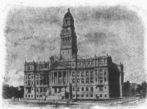
WAYNE COUNTY BUILDING, DETROIT.
