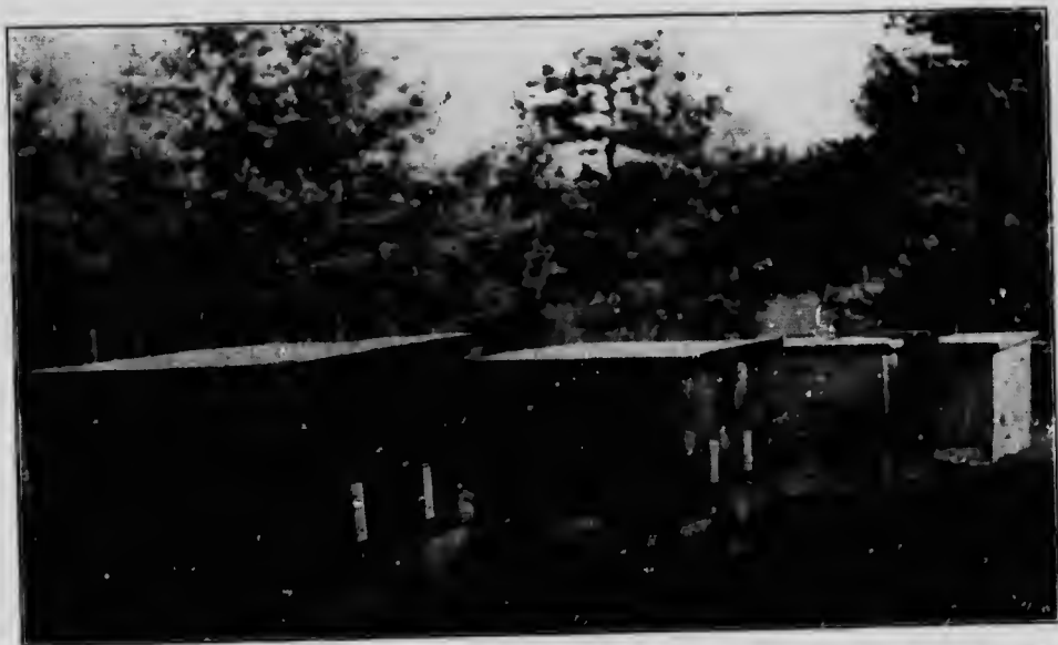
Row of quadruple cases with entrance doors open as in warm weather of spring or fall. These doors close \frac{3}{8} -inch short of ends of openings leaving winter entrances \frac{3}{8} -inch wide by 1\frac{1}{2} inches high.
