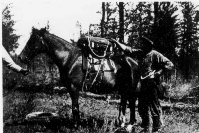
Fig. 6 Mobley wire-craddle as used with one coil
