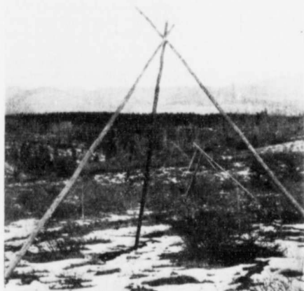
Fig. 19 Tripod line supports
