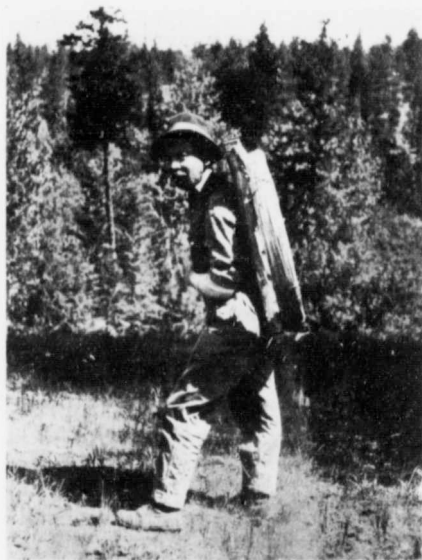
Fig. 8 Klondike pack-frame as used for packing wire
