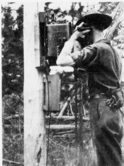
Fig. 48. Lookout station telephone set installed in the field
