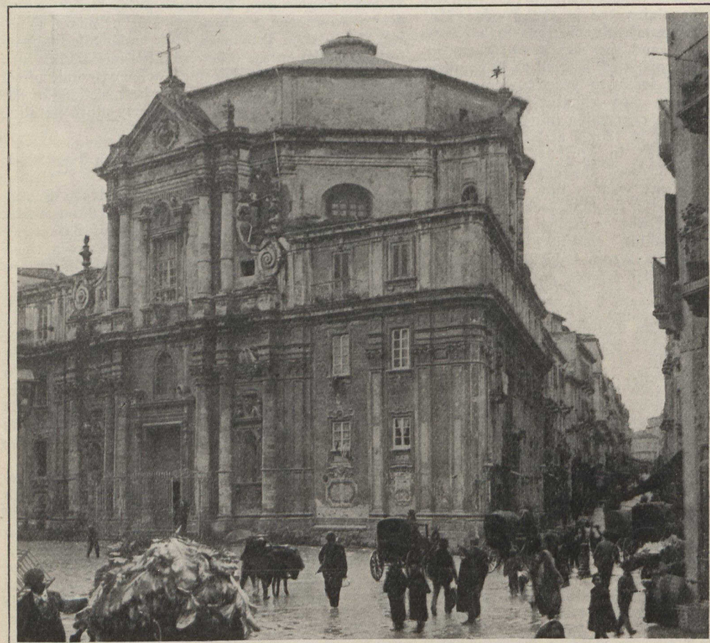
Church of the Souls in Purgatory, Messina, which gives some idea of the beauty of the ancient buildings which added charm to the one-time smiling seaport.
