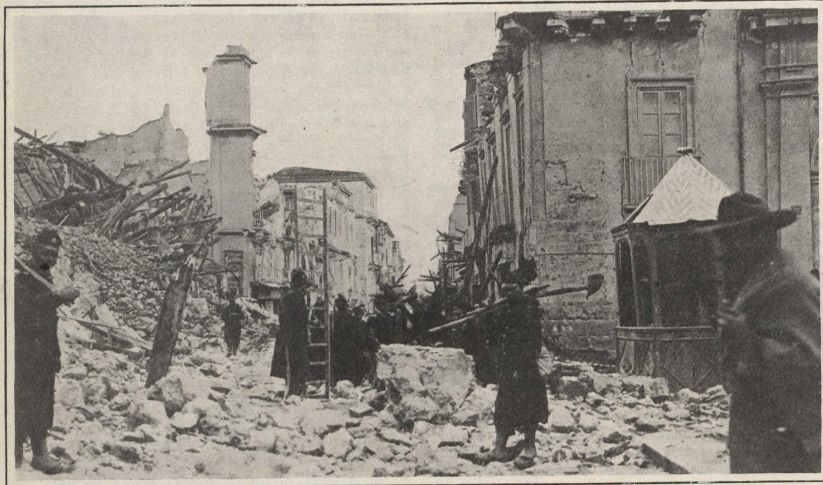
This gives a vivid picture of the wrecked houses and other buildings. The debris-covered streets indicate how small was the chance of escape.
