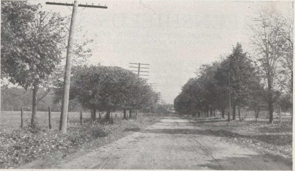
A mile of trees "shorn" to allow of the passage of wires. As thousands of stubs have been left, nearly every tree will die. In winter the effect of "shearing" is horrible. Co-operation will largely prevent such mutilation in the future.
