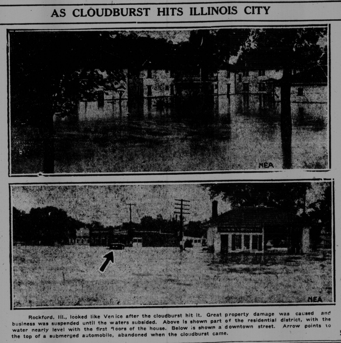
Rockford, Ill., looked like Venice after the cloudburst hit it. Great property damage was caused and business was suspended until the waters subsided. Above is shown part of the residential district, with the water nearly level with the first floors of the houses. Below is shown a downtown street. Arrow points to the top of a submerged automobile, abandoned when the cloudburst came.
