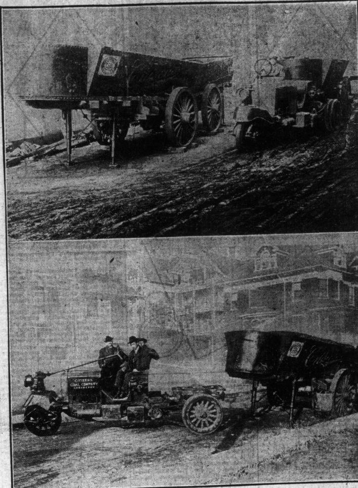
PHOTOGRAPH SHOWING HOW THE KNOX MARTIN TRACTOR IS USED WITH INTERCHANGEABLE BODIES, ENABLING THE TRACTOR TO BE KEPT CONSTANTLY AT WORK WITH A HIGH EARNESTING CAPACITY.
