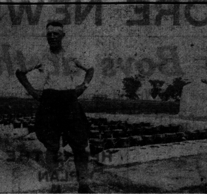
Cook-Sergeant Nixon of the 180th Battalion standing in front of his Aldershot kitchen. There are 99 kettles in the kitchen, each holding enough soup for 15 men. The kettles are set in clay molds, built on the ground, with flues running to the chimney in the rear.
