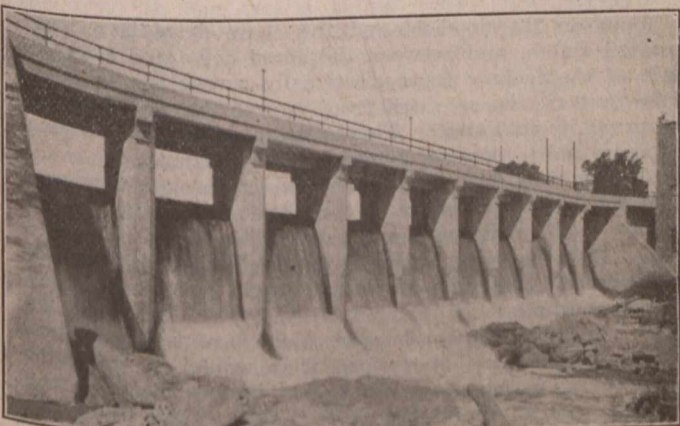
FIG. 2—A CLOSER VIEW OF THE DAM
