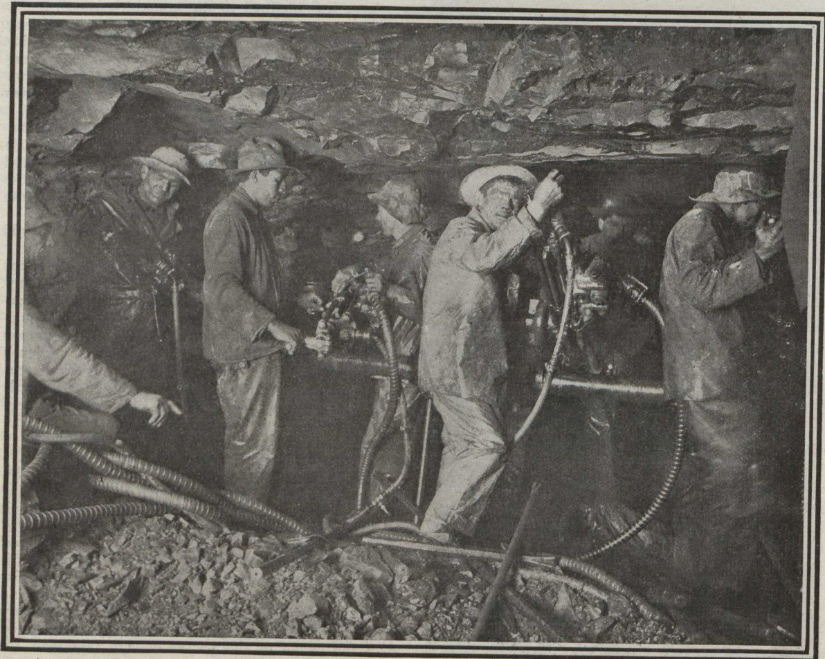
Heading from the West in the Great Railway Tunnel Through Montreal Mountain.
