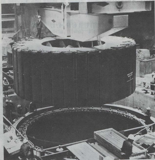
Two powerhouse cranes, with a combined lifting capacity of 800 tons, have been responsible for the placement in the machine hall of such pieces of equipment as the rotor and alternator pictured here. With a diameter of 30 feet and a height of close to 10 feet, the rotor of each of the 11 generating units at Churchill Falls weighs 650 tons.
