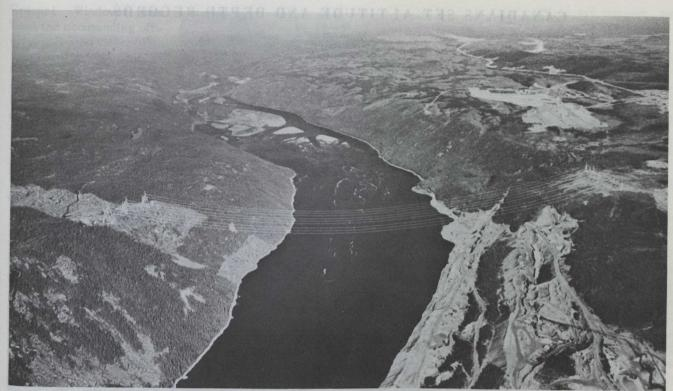
In July 1971, 36 strands of subconductors were pulleyed across the Churchill River to complete one of the more graceful phases of the hydro-electric power development at Churchill Falls. The strands
