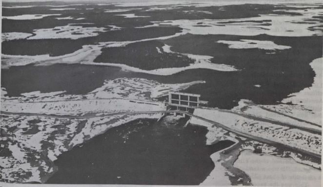
The control structure at Lobstick regulates the flow of water from the Smallwood Reservoir to the forebay. Once full, the Smallwood Reservoir (shown behind the Lobstick structure) will provide the powerhouse with a potential
