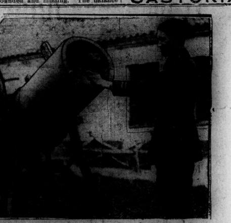
**TRENCH MORTAR CAPTURED BY THE CANADIANS.** — It is made of wood and bound with wire.
