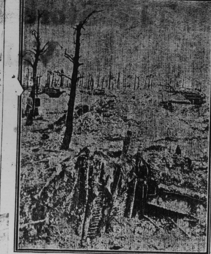
WHEN BIG GUNS HAVE DONE THEIR WORK. German defences leveled by shell fire in preparation for an infantry assault. Naturally nothing could stand up under such an avalanche of fire. (London Mirror photo.)
